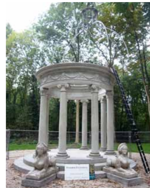
The dome is also a very important piece of art history. It is regarded as a folly: a whimsical, artistic structure with no purpose except to decorate the surroundings and offer a place to rest for a while.
