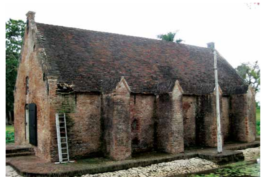
Kruithuis Built in 1778, this is a typical Dutch building that is a very fitting part of a fort.
